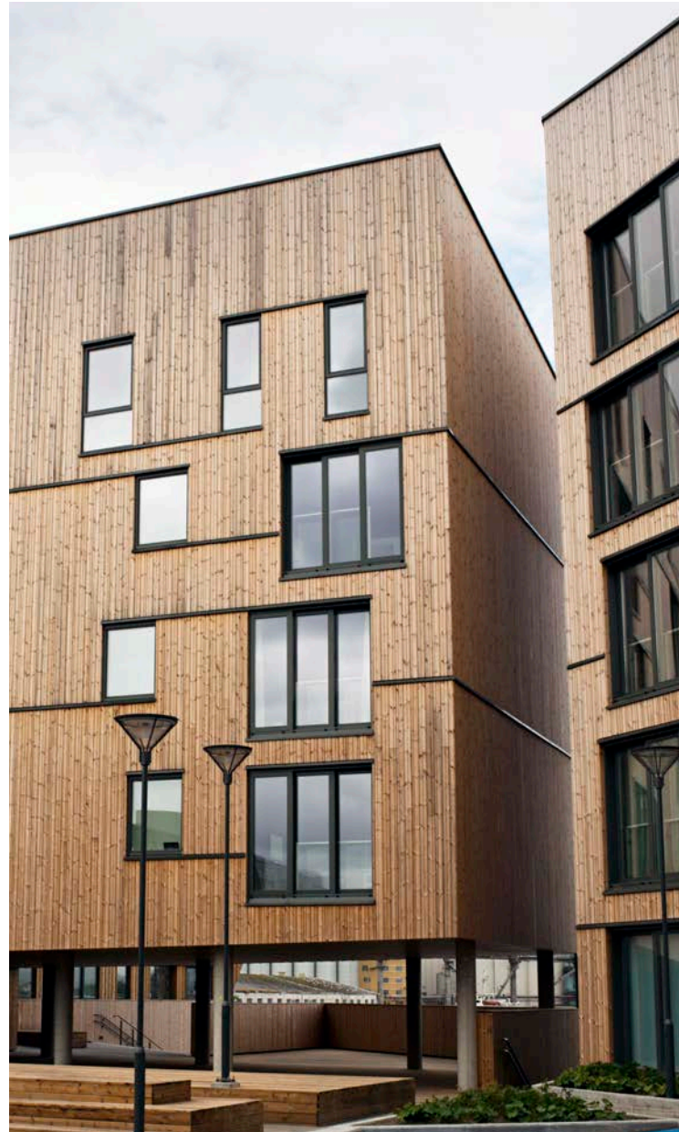
Vannkanten i Stavanger, AART Architects
